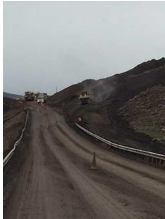
Crews work to expand the width of the highway
